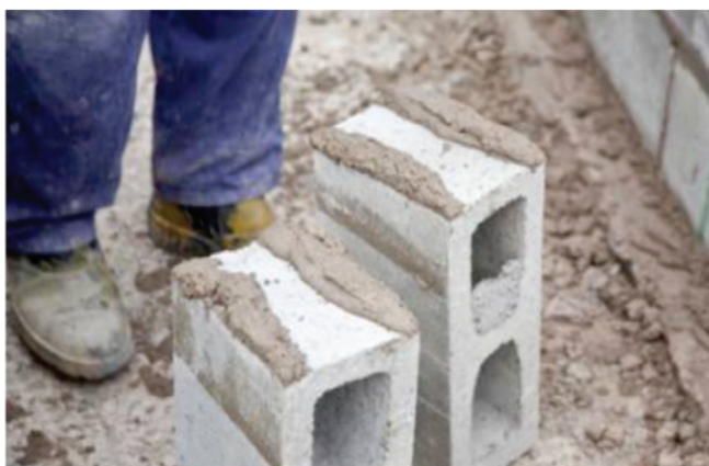
Argamassa na vertical
